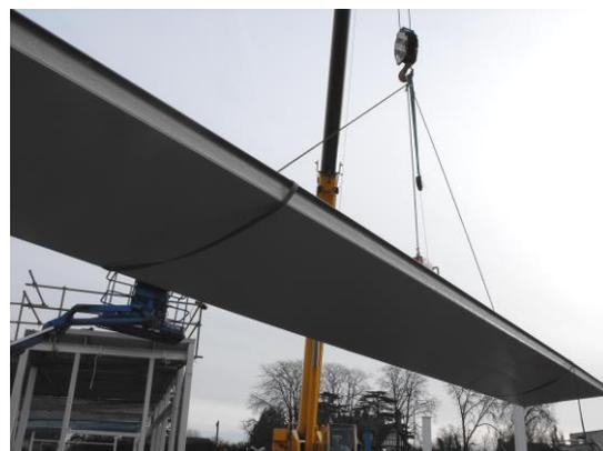
The Clad Boy® is a proven vacuum panel lifter and many installers are familiar with this type of equipment. With internal re-chargeable battery power, the Clad Boy® enables rapid panel installation rates, taking advantage of the 2m cover width provided by the KS2000RW panel.
