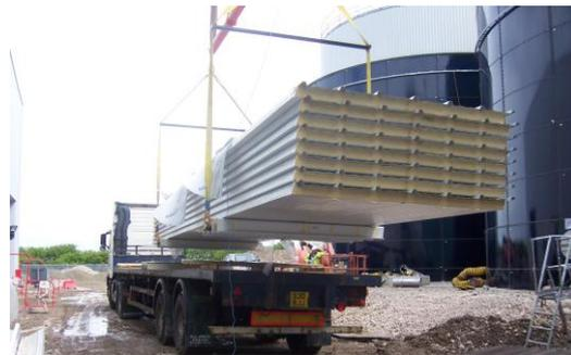
Various Pack Boy™ kits are available and the range is flexible to allow adaptation to suit all pack sizes. The maximum allowable pack weight for any single Pack Boy™ system is 5 tonnes. All users must take the weight and effective working height of the Pack Boy™ kit into account when sizing cranes – full details are provided on the panel off-loading chart.
