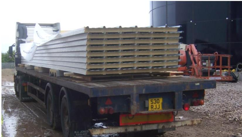
The purpose of the X-dek bearers is to allow un-loading beams to pass through the bearers and the locations of the bearers are agreed with Kingspan to suit the Pack Boy™ modular off-loading system. Refer to the separate chart detailing Pack Boy™ beam centres, lifting capacities and lift heights for details.
