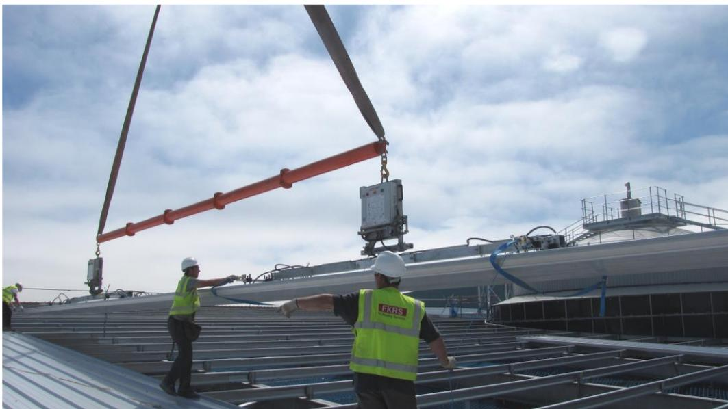
This impressive system has already been used to handle panels up to 21m long and has the capability of lifting 24m panels with ease.
