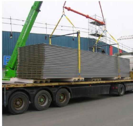
For Panel Lengths Over 15 metres up to 20 metres, 4 Lifting Points
