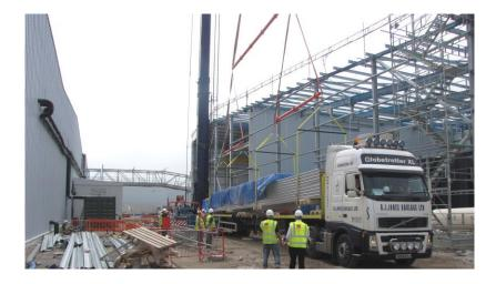
If you intend to use the Pack Boy<sup>TM</sup> system to off-load the panels it is imperative that Kingspan are notified at the earliest possible moment to ensure that the packs are suitably arranged.
