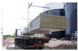
Various Pack Boy<sup>TM</sup> kits are available and the range is flexible to allow adaptation to suit all pack sizes. The maximum allowable pack weight for any single Pack Boy<sup>TM</sup> system is 5 tonnes. All users must take the weight and effective working height of the Pack Boy<sup>TM</sup> kit into account when sizing cranes – full details are provided on the panel off-loading chart.
