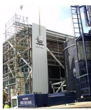
Due to the size and weight of the panels this technique is most suitable for use with cranes rather than telehandlers of forklifts. It should also be noted that the large surface area of the panel will increase susceptibility to wind loading and lower wind limits may therefore apply.
